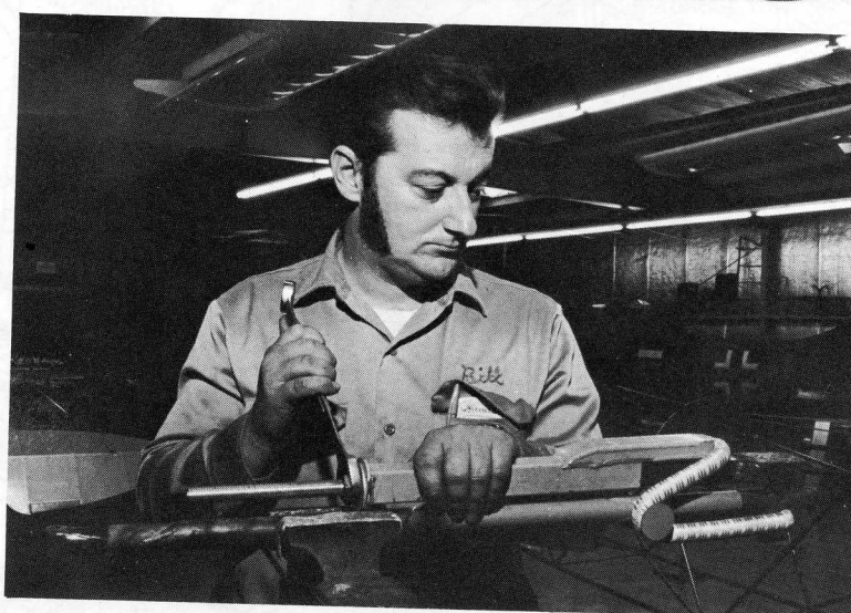
Putting shock cord in place with landing gear shock strut.
